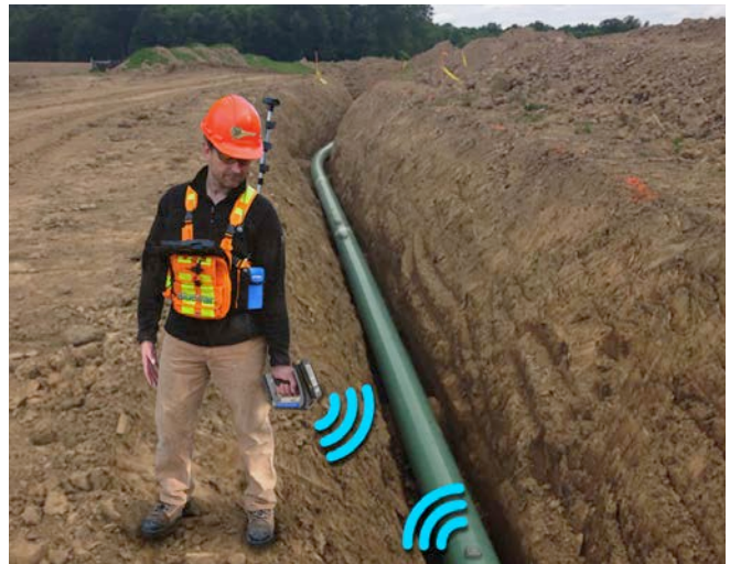
Figure 4. Confirming the data prior to backfilling by reading the RFID tag.
