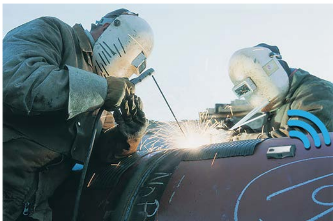
Figure 3. RFID tag is captured in the weld log to ensure data integrity.
