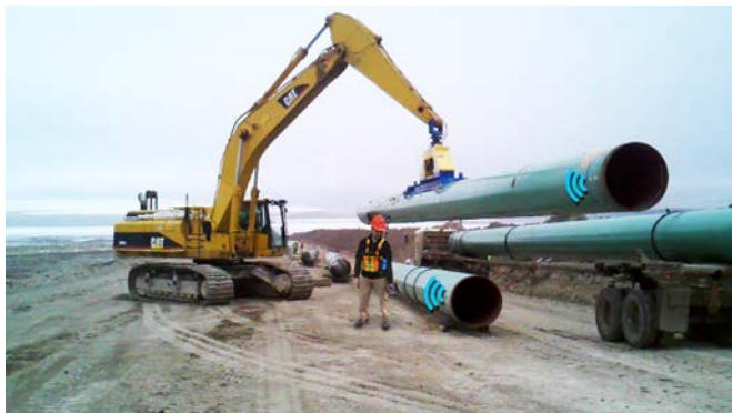
Figure 2. Registering the location when stringing pipe using RFID coupled to GPS.
